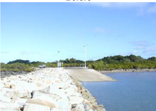
Finished Rock Wall
